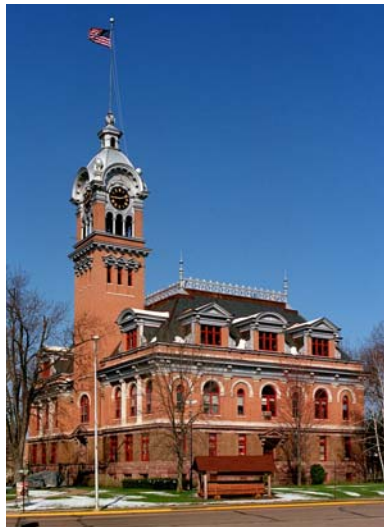
After 22 years of debate, the Lincoln County Courthouse – one of Wisconsin’s historic gems – will be expanded.
